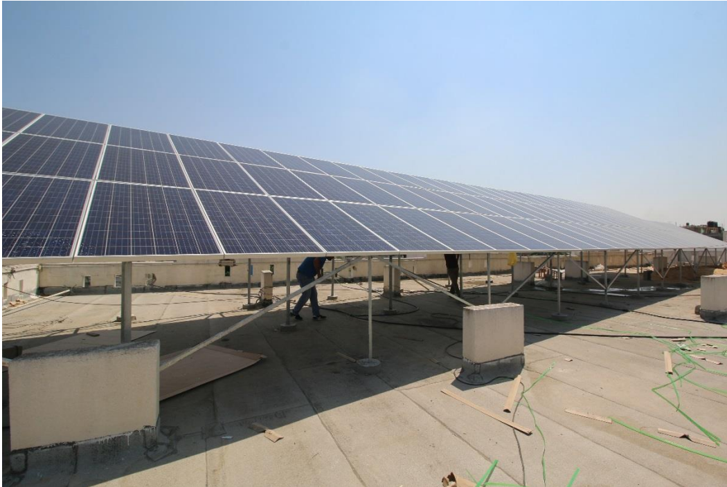
Figure 11: Solar Panels just installed on the top of Beit Hanoun Hospital
